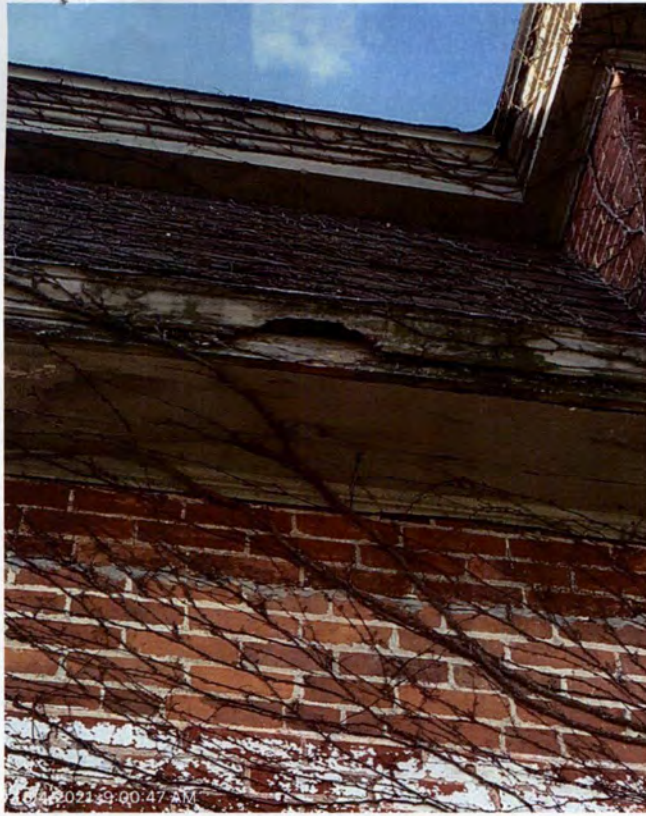
Deteriorating trim at rear of property
