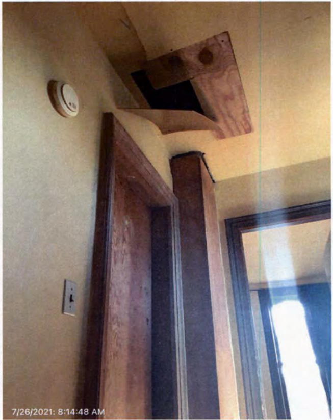
Collapsing ceiling in front entryway
