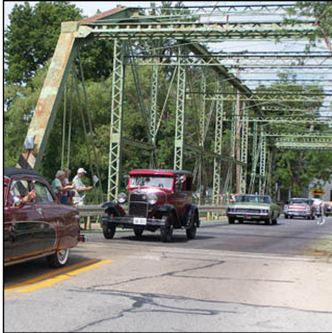
INDIANA AVENUE BRIDGE aka. Historic "Fort Wayne Street Bridge"
